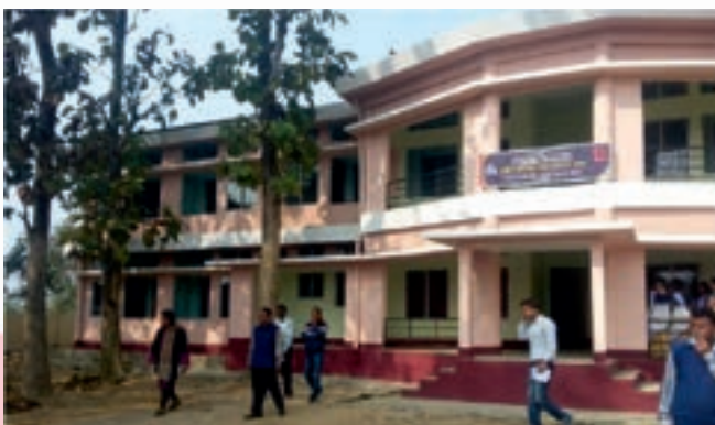
Newly constructed Girls Hostel, KGBV (Type-IV)
