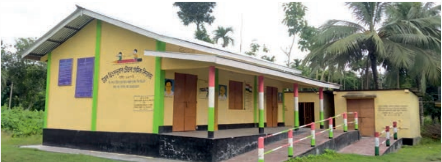
Additional classroom in school
