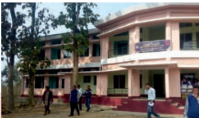
Newly constructed Girls Hostel, KGBV (Type-IV)
