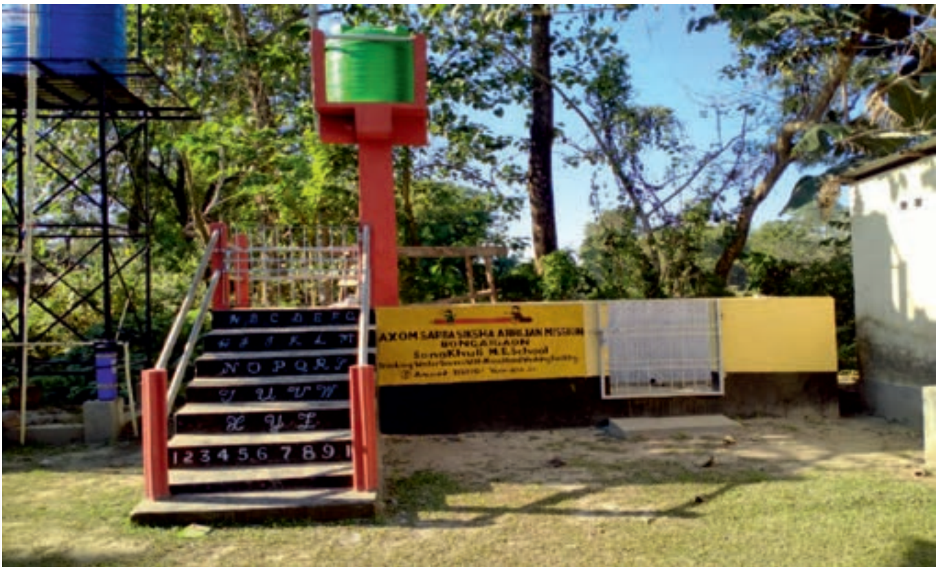
Drinking water facility in school
