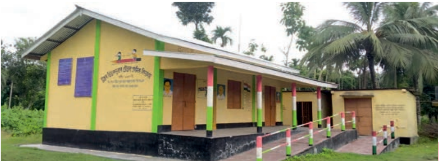
Additional classroom in school
