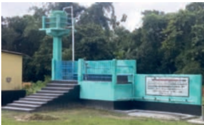
Drinking water facility in school
